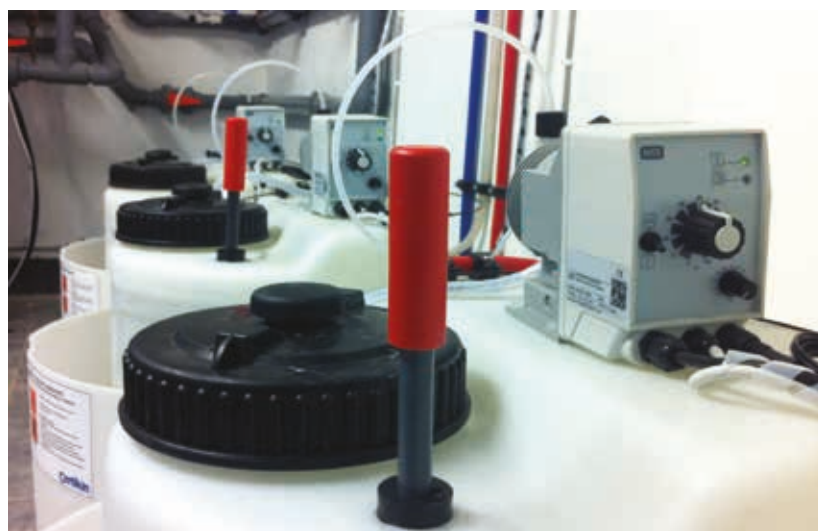
Example pump, tank and bund set fitted with a manual mixer
