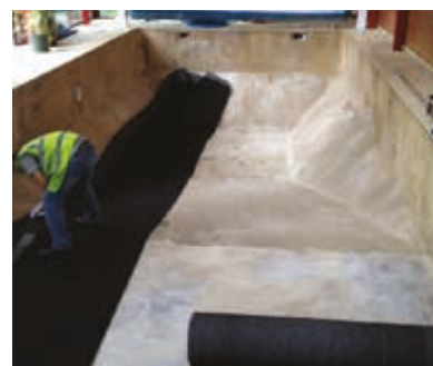
Liner underlay for bag & site lined pools
